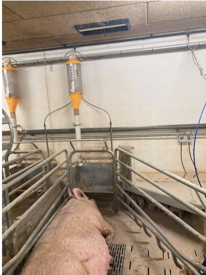
Ventilation is provided above each sow
