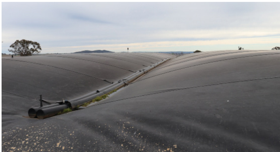
Figure 13.2 Unheated and unmixed covered anaerobic pond
