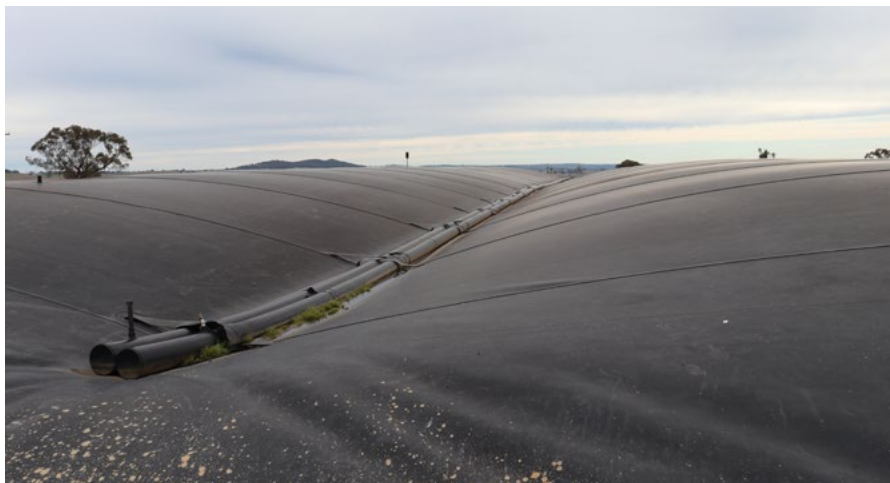
Figure 13.2 Unheated and unmixed covered anaerobic pond
