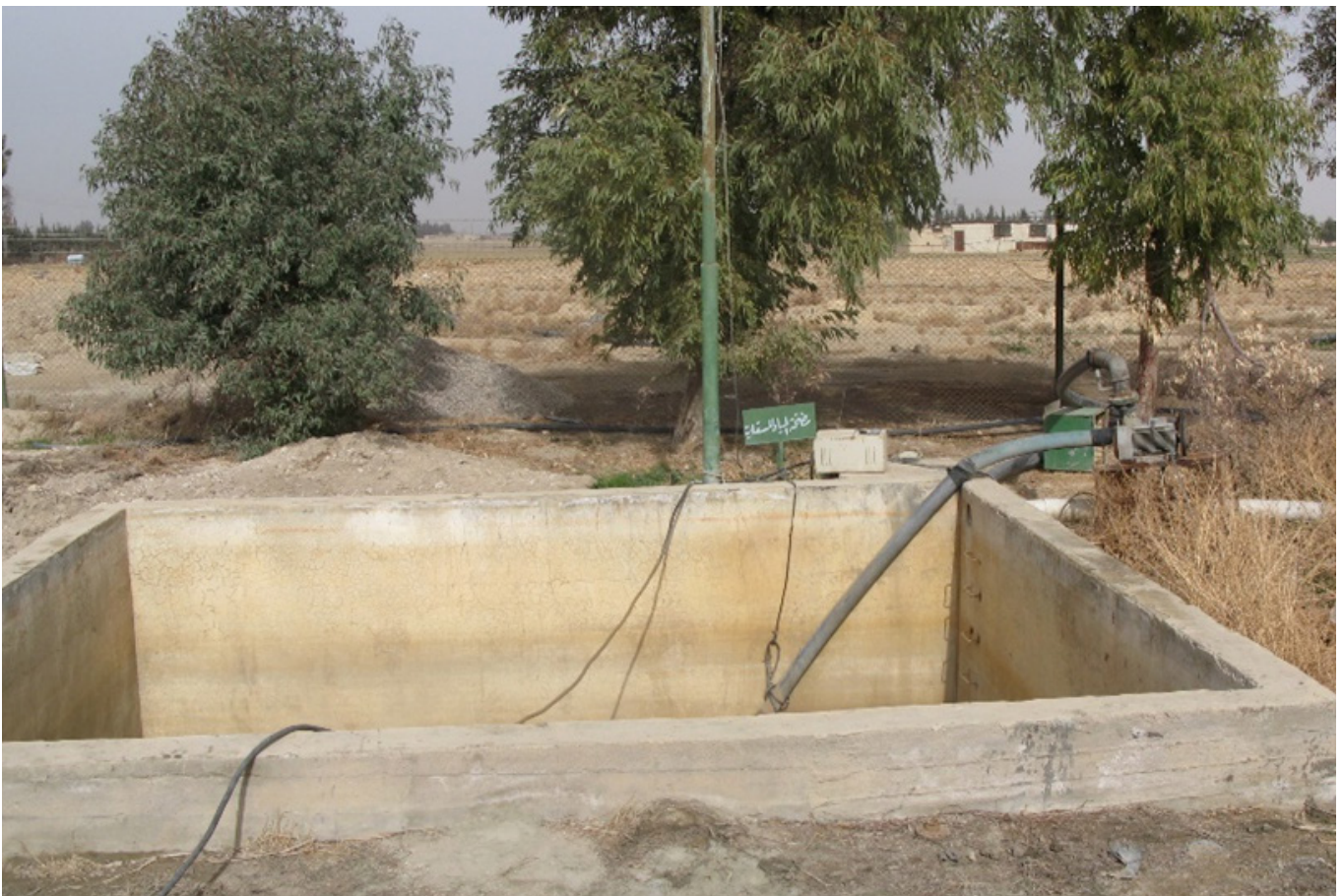
Figure 1. Square effluent storage tank
