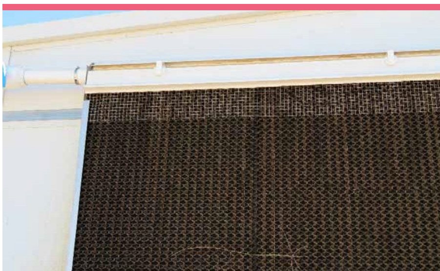
Figure 1. Small gauge wire (< 5mm) can exclude rodents.
