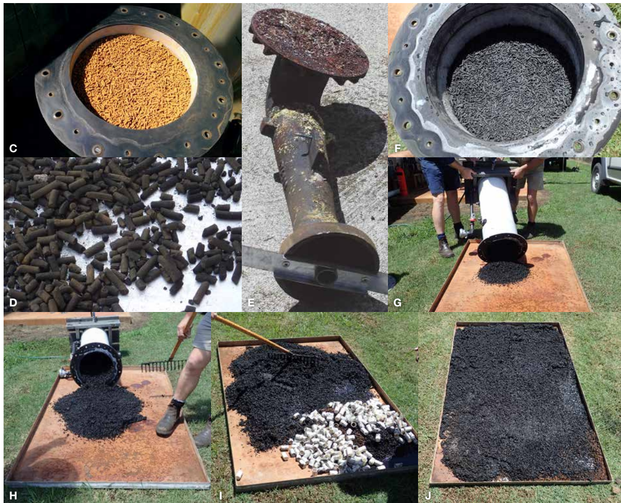
FIGURE Biogas infrastructure at Case Study 5 piggery
