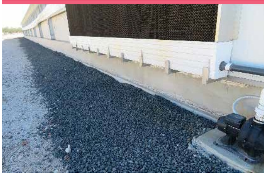
Figure 2. An example of compacted road base along shed parameters to prevent rodents burrowing.
