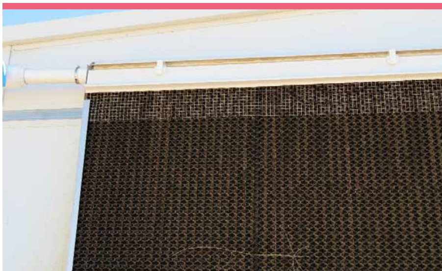
Figure 1. Small gauge wire (< 5mm) can exclude rodents.
