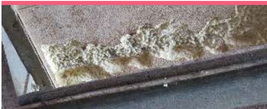
Figure 4. Damage to insulation caused by rats.
