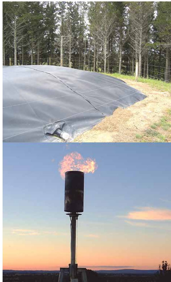
FIGURE An impermeable lagoon cover at a New Zealand piggery. An impermeable cover provides a gas-tight seal that captures biogas and emitted odour. When biogas is burnt in a flare, onsite generator or hotwater system, odorants in the biogas are destroyed.
