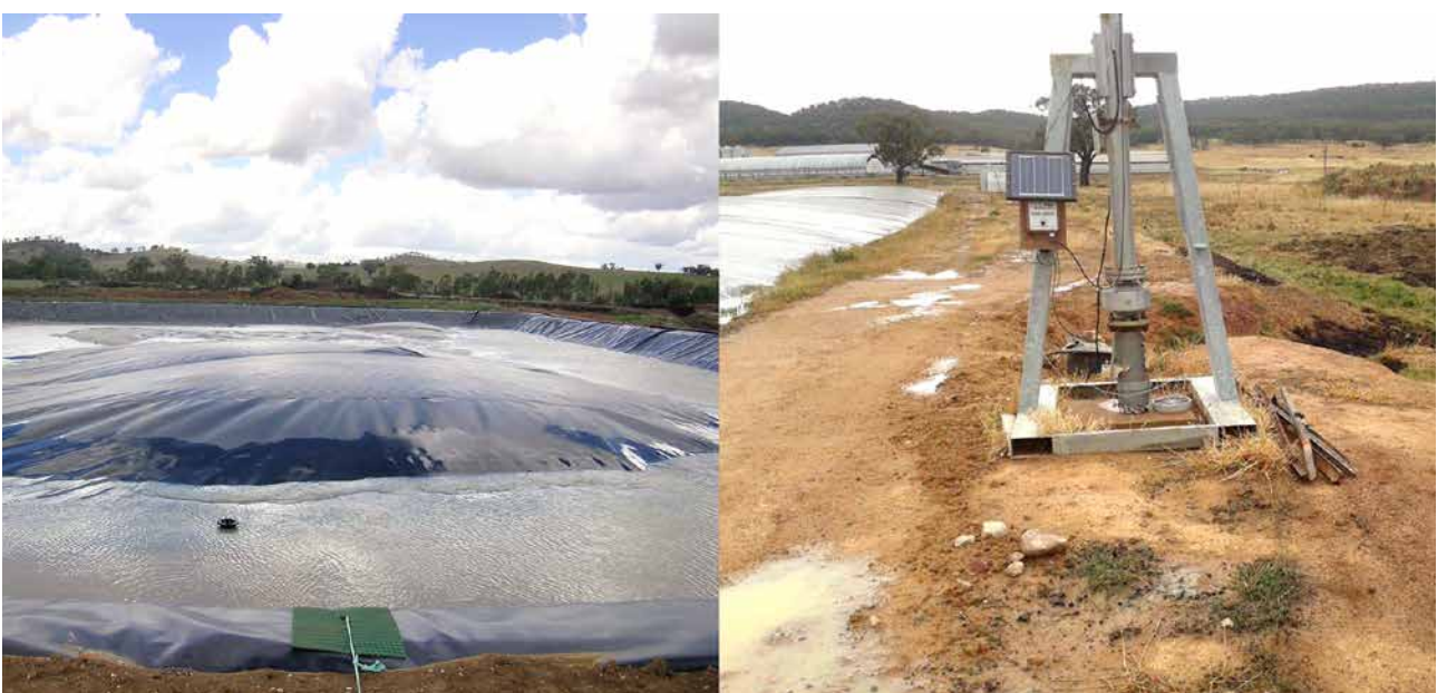
FIGURE 4 Stormwater and related management with covered lagoons at Australian piggeries. (Left) Unwanted, a biogas whaleback trapped by a rim of stormwater; (Right) Wanted, a fire break with regularly maintained vegetation around the lagoon perimeter prevented a bush fire from progressing up to the cover before it was extinguished.
