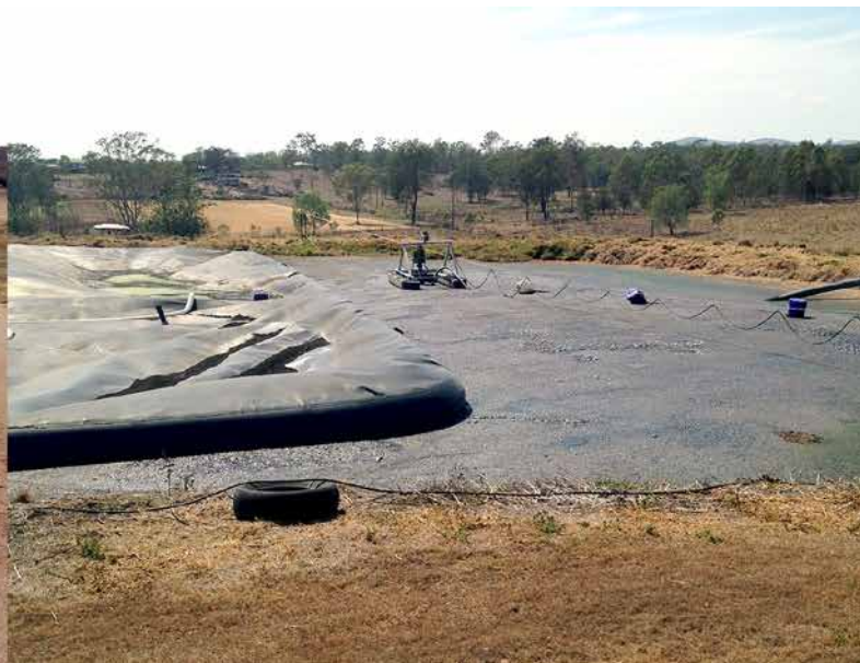
FIGURE 2 Floating hood covered lagoon arrangement at an Australian piggery
