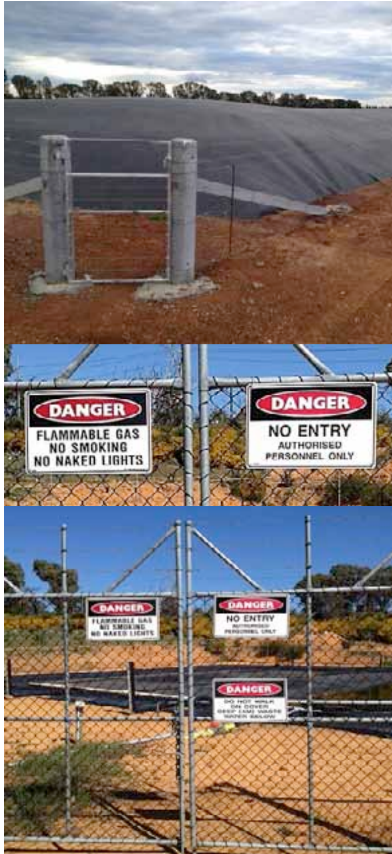
FIGURE 5 Fence exclusion can clearly mark restricted access areas and related hazards
