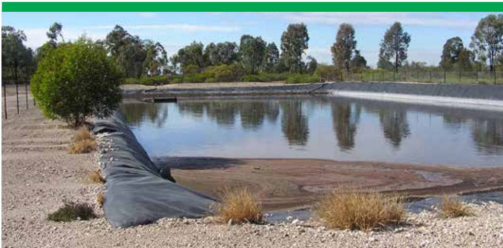
Photograph 11 Plastic lined anaerobic pond
