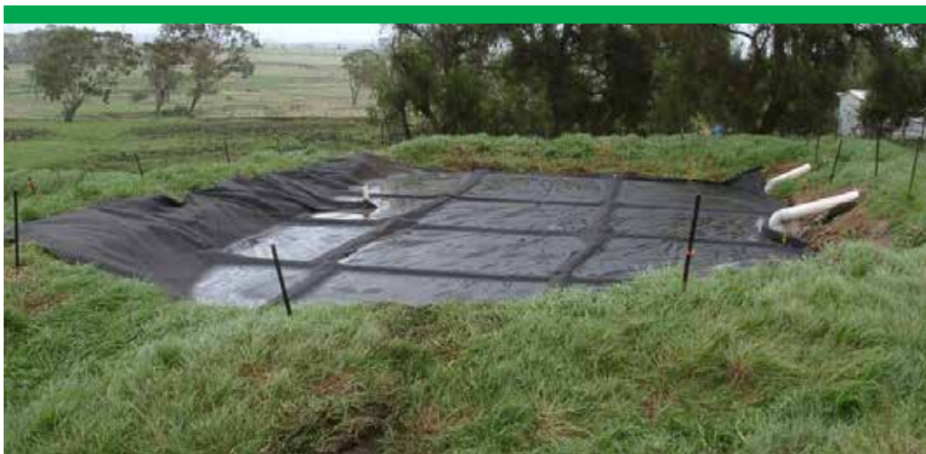
Photograph 14 Semi-permeable pond cover
