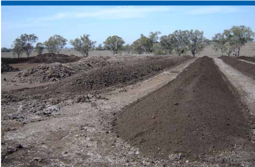
Photograph 27 Sloping sides on windrows promote shedding of water
