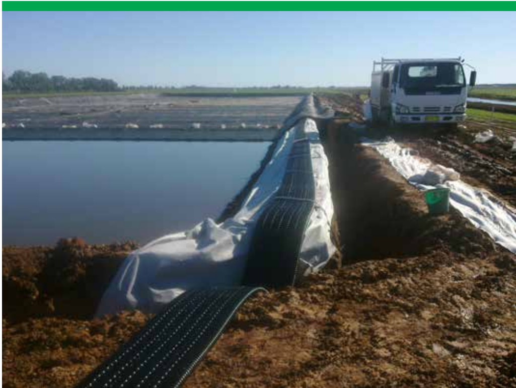
Photograph 15 Covering a piggery effluent treatment pond
