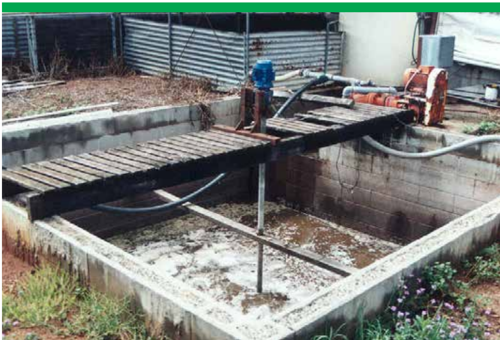
Photograph 6 Effluent collection sump
