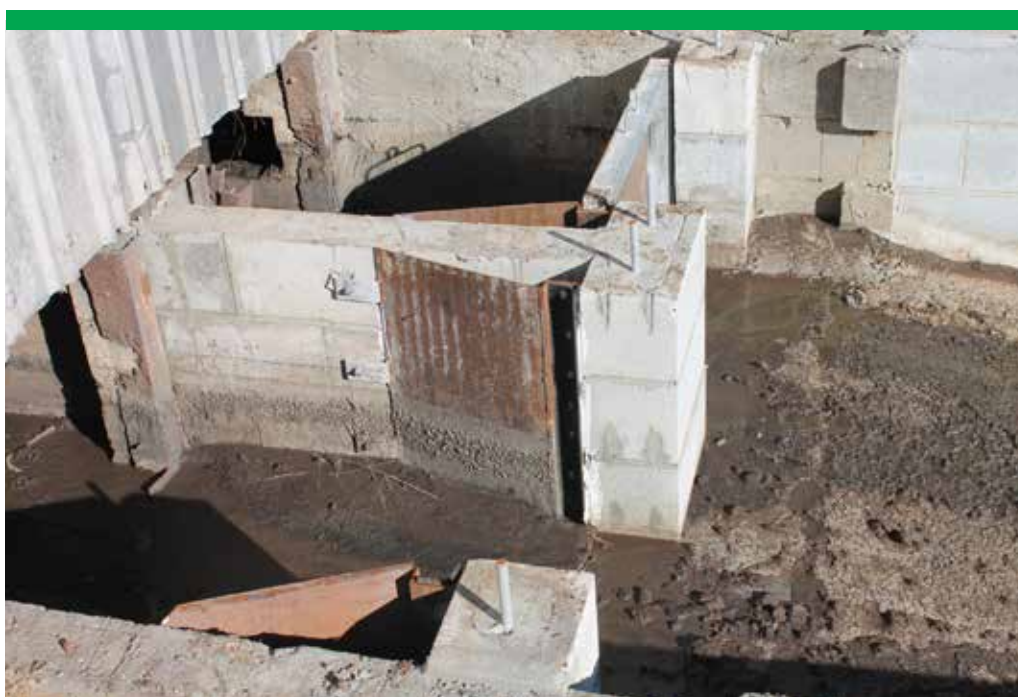
Photograph 5 Sluice gates on a static pit
