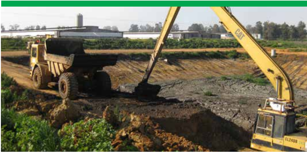
Photograph 20 Sludge removal with a long-reach excavator
