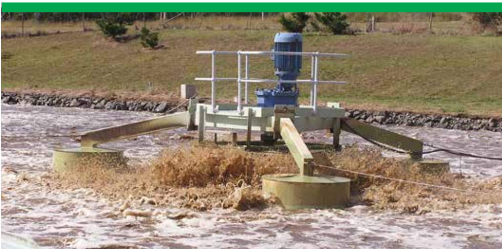
Photograph 19 Aerator on surface of pond
