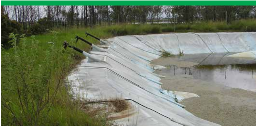
Photograph 24 Sludge extraction pipelines (deflated pond cover)
