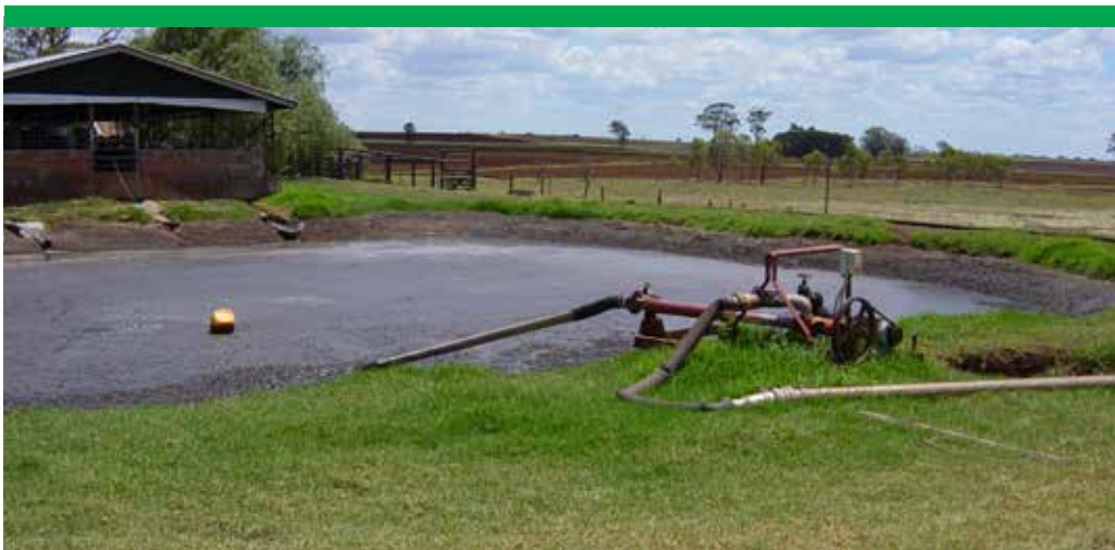
Photograph 21 Sludge removal with a Mono-Pump
