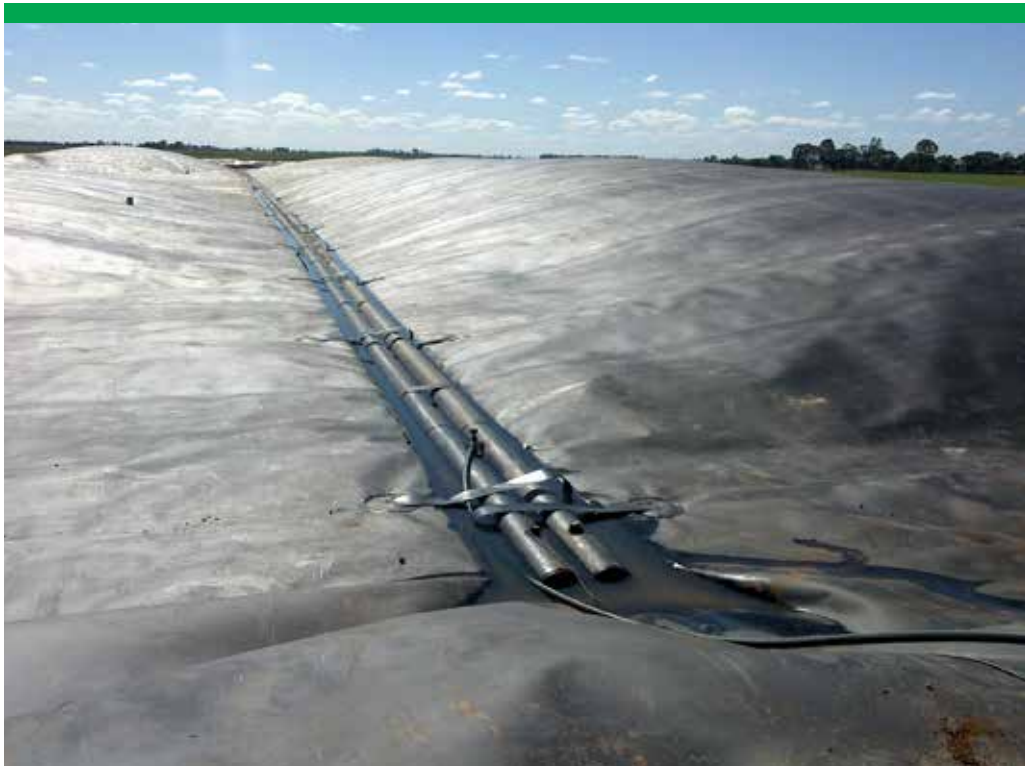
Photograph 16 Covered anaerobic pond with weight pipes installed on cover
