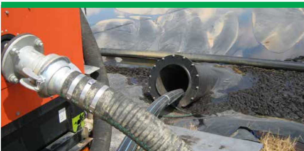
Photograph 25 Pump suction pipe inserted into in-situ desludging pipe
