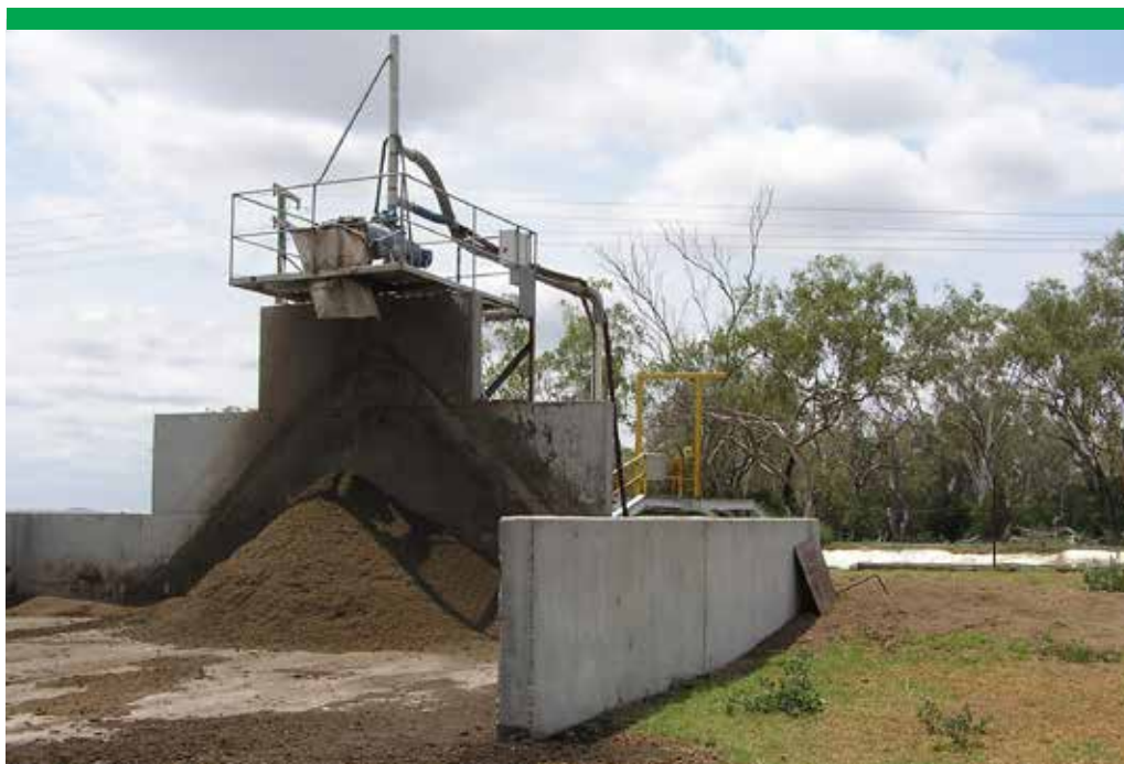
Photograph 8 Screw press separator
