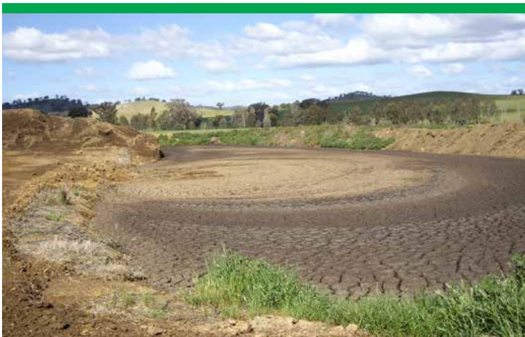
Photograph 26 Sludge drying bay
