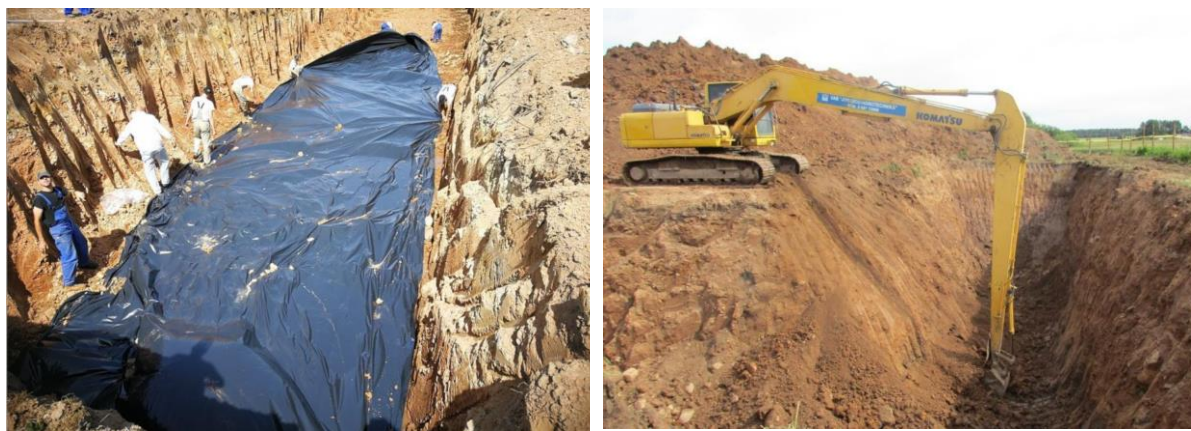
Figure 23. On-farm burial trenches in Lithuania – with lining on the left. Source: Paulius Busauskas
