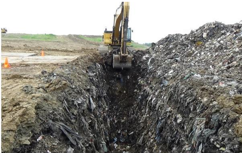
Figure 26: Trenching within existing waste cell. This example photo was taken during a HPAI response in the USA. (Courtesy of USDA-APHIS).
