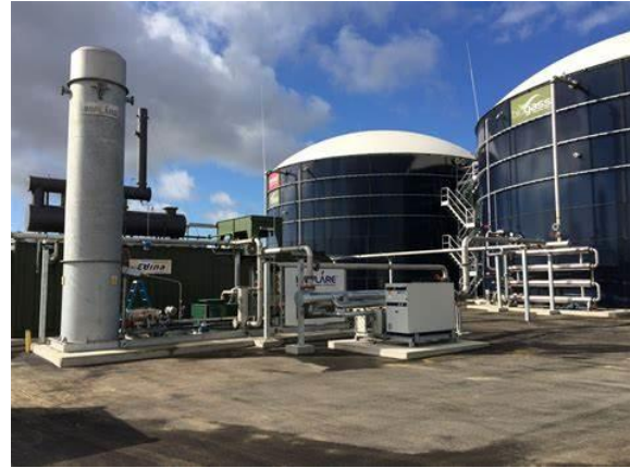
Figure 35: Anaerobic digester tanks
