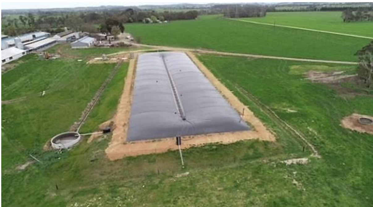
Figure 2 Photograph of onsite covered anaerobic pond at the biogas case study piggyery. The pond is approximately 25m wide, 100m long and 5m deep with an internal batter slope 1:2 (vertical:horizontal). Liquid treatment volume is approximately 5.5ML including sludge storage. Total pond volume is approximately 6.5ML. Typical operating freeboard is approximately 0.5m. The pond cover can provide additional gas storage for an estimated 2,300m 3 @ 50Pa.
