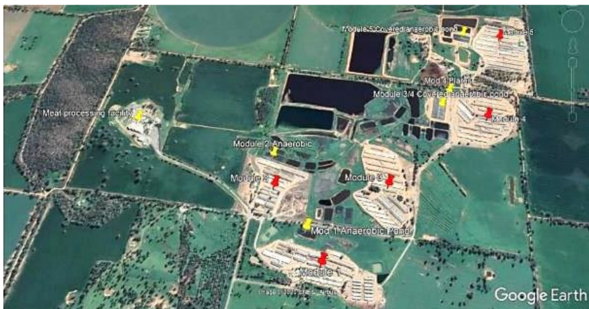
Figure 10 Aerial Photograph of large Australian piggery that voluntarily participated in the biomethane study, showing various biogas components onsite at the piggery
