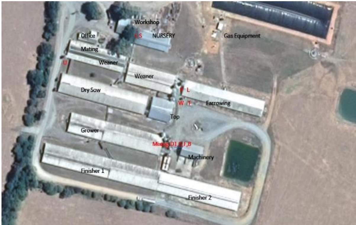
Figure 1 Aerial photograph of biogas case study piggyery, showing shed layout. The covered pond and biogas equipment are visible in the top right-hand corner.
