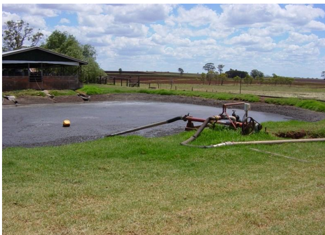
Figure 1: Sludge removal via pumping
