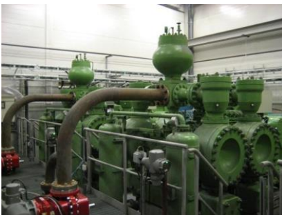
Figure 4: Heavy duty industrial GEHO PD - ZPM Pump
