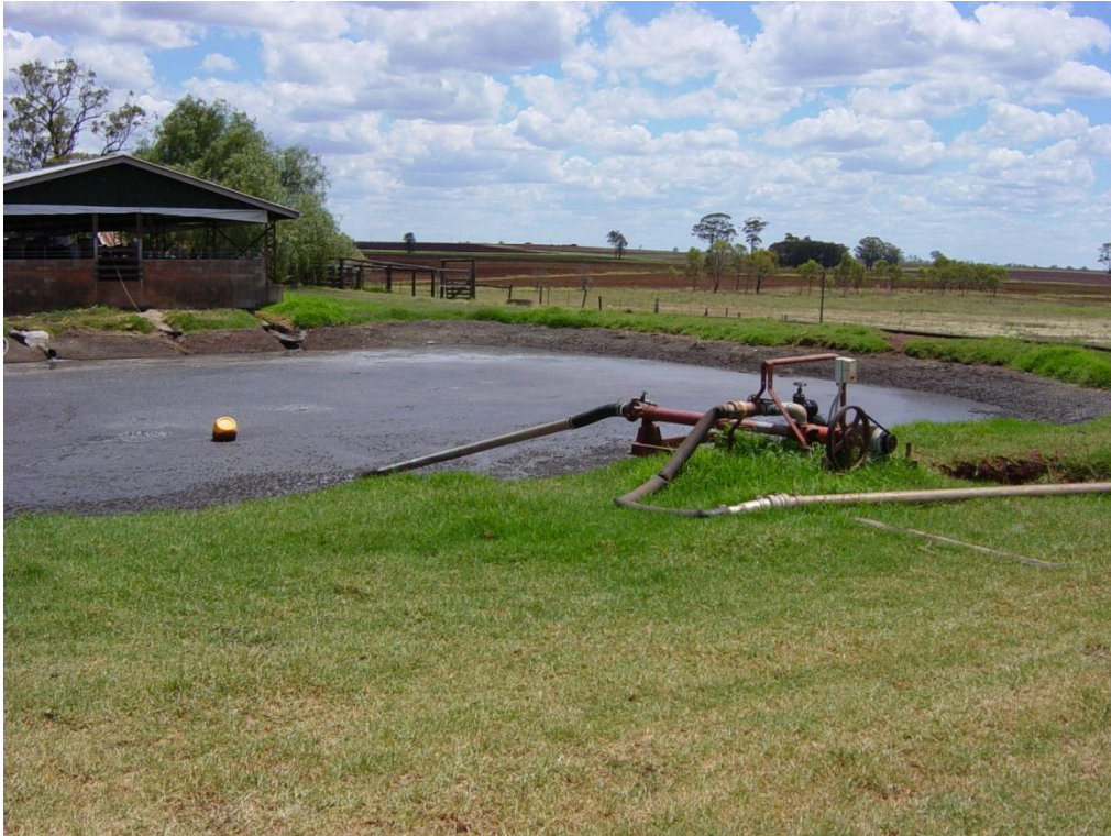
Photograph 9: Sludge removal with a mono pump (no agitation)
