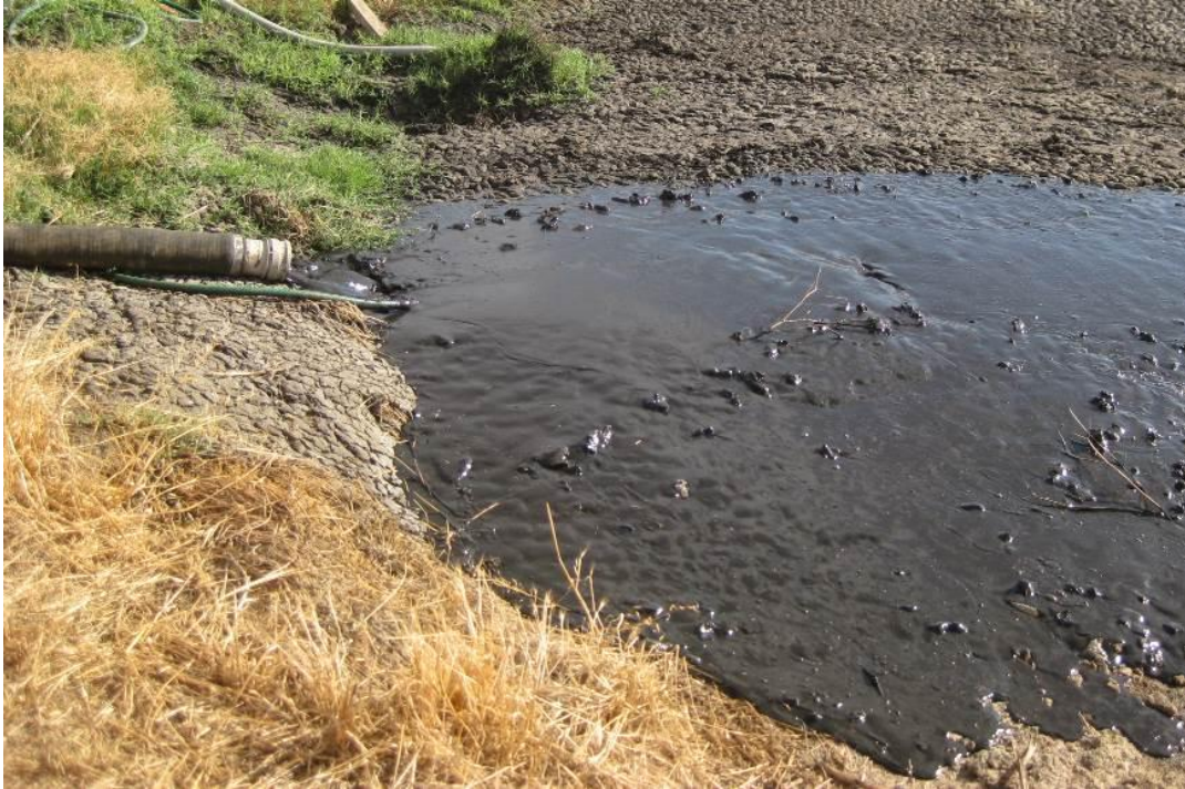
Photograph 44: Sludge removed from CAP during pump priming
