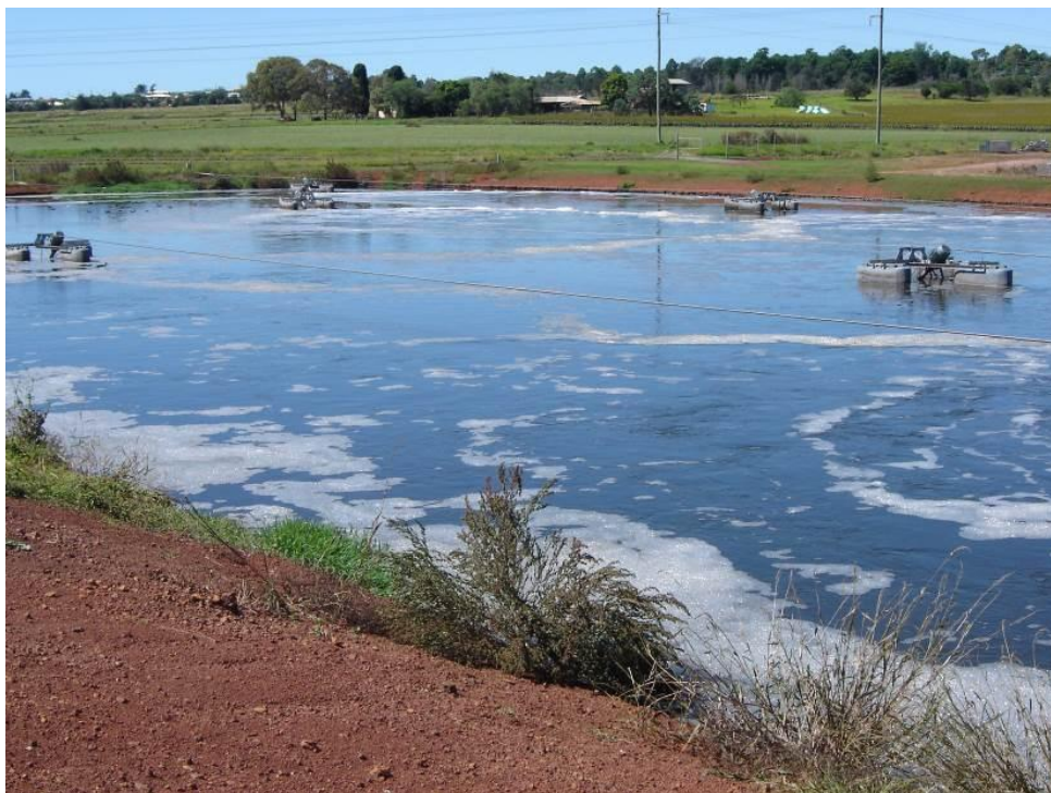
Photograph 4: Mechanically-Aerated Aerobic Pond
