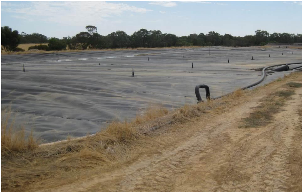
Photograph 1: Covered anaerobic pond
