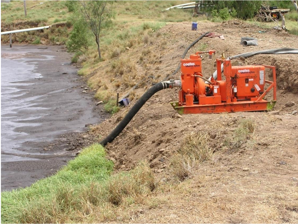
Photograph 5: Dewatering an anaerobic pond prior to desludging
