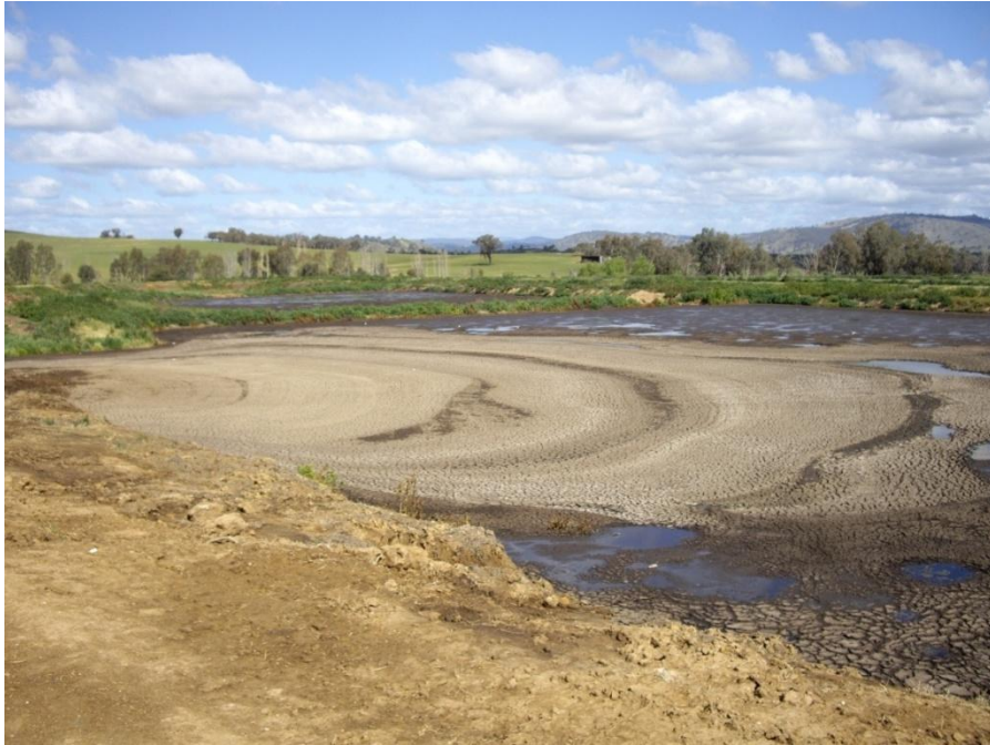
Photograph 19: Long-term sludge drying bay
