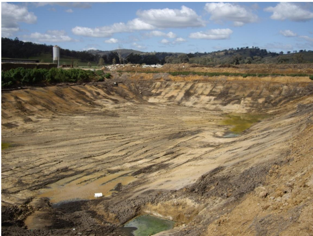
Photograph 8: Anaerobic pond after dewatering and desludging
