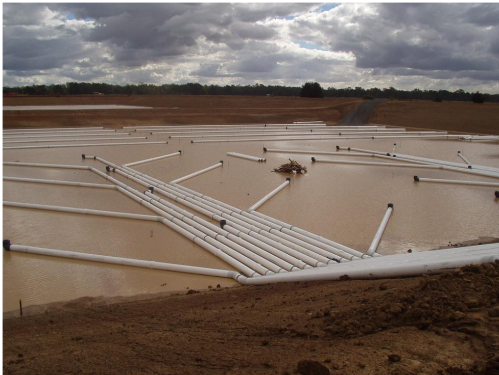
Photograph 15: Installation of sludge removal pipe system
