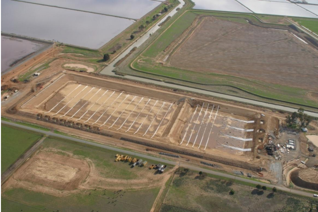
Photograph 14: Installation of sludge removal pipe system
