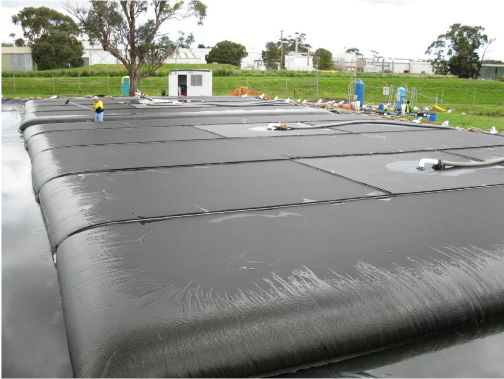
Photograph 26: Dewatering sludge using geotextile tubes (Dredging Solutions)
