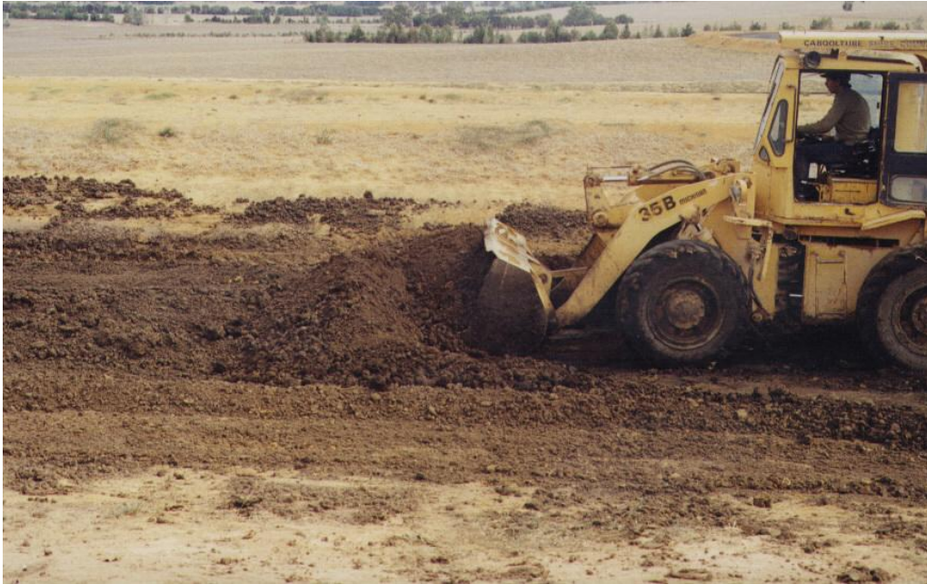
Photograph 24: Solids removal from dried SEPS bay
