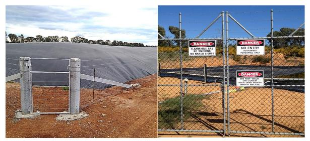
Figure 2.1 Fence exclusion can clearly demarkate restricted access areas and related hazards (Photos courtesy of the Pork CRC)
