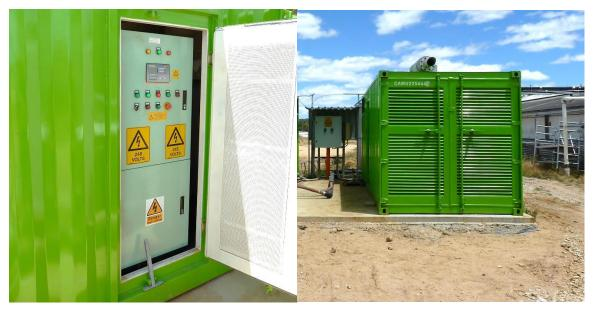
Figure 2.4 Emergency switches located outside an on-farm generator skid (Photos courtesy of the Pork CRC)
