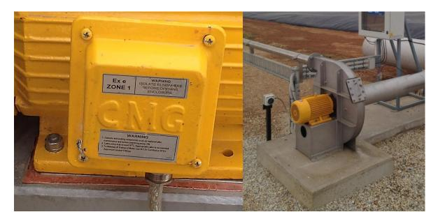
Figure 2.2 Example of a biogas blower at an Australian piggery rated to Zone I (Photos courtesy of the Pork CRC)
