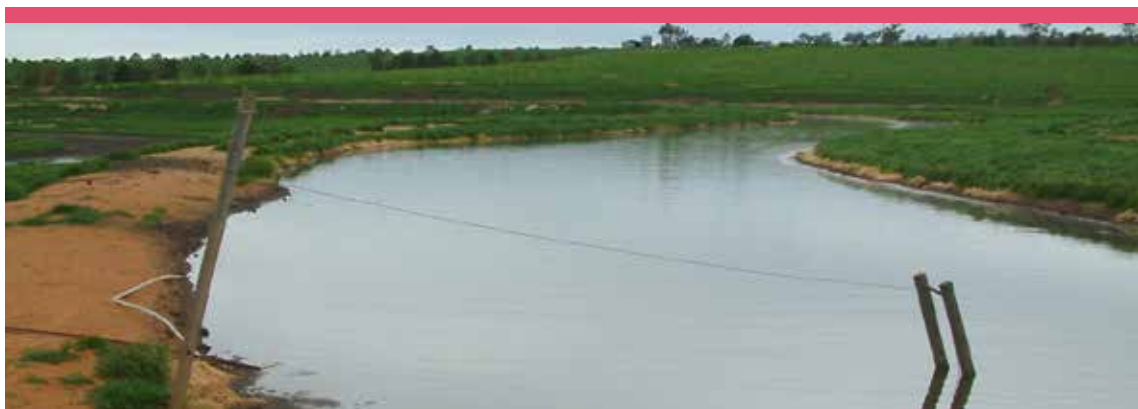
Photograph 5 Raised syphon pipe on simple winch at exit end of SEPS channel
