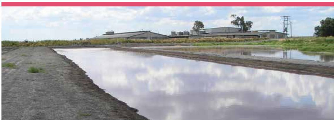
Photograph 4 SEPS channel on flat site (photo courtesy of Alan Skerman)
