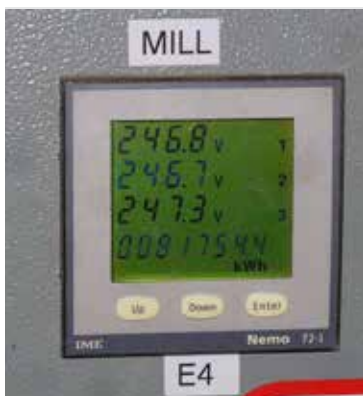
Photograph 6 Solid State Power Meter Showing the Voltage of Each Phase and the Power Usage
