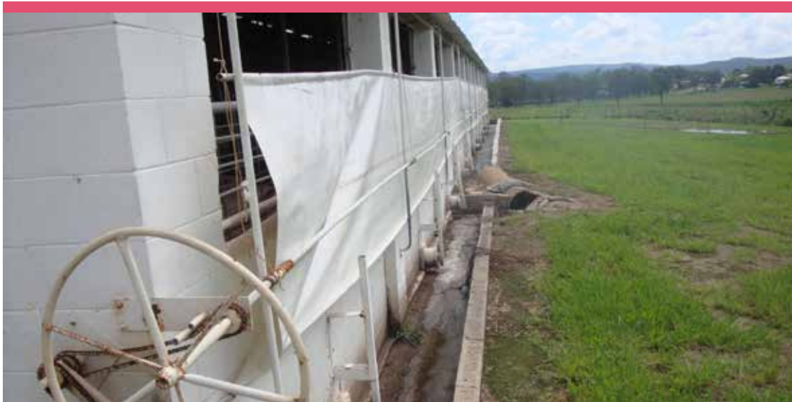
Photograph 3 Naturally Ventilated Shed
