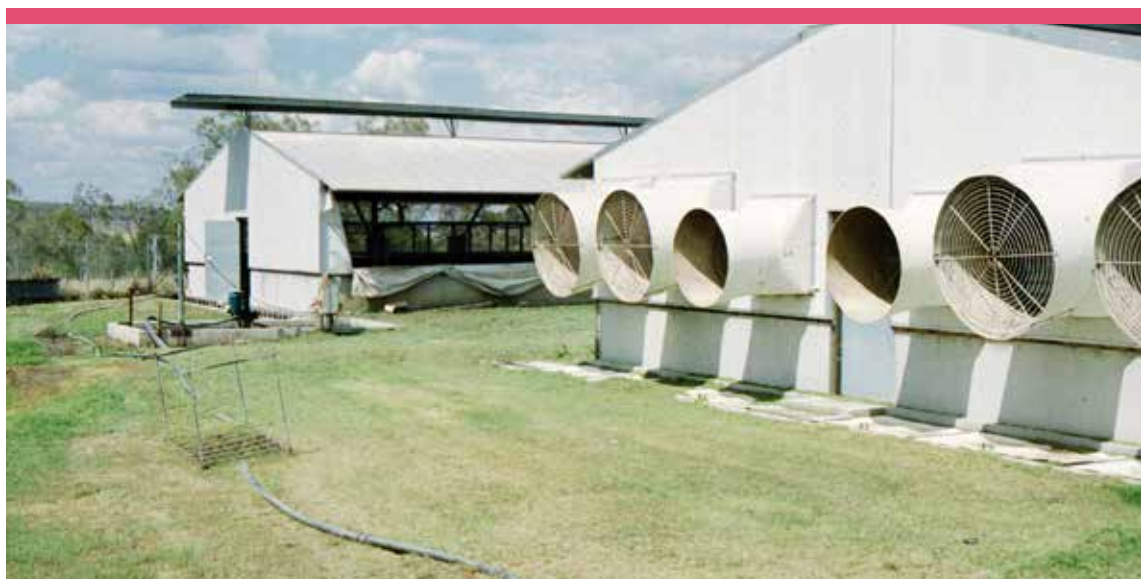
Photograph 2 Tunnel Ventilated Shed
