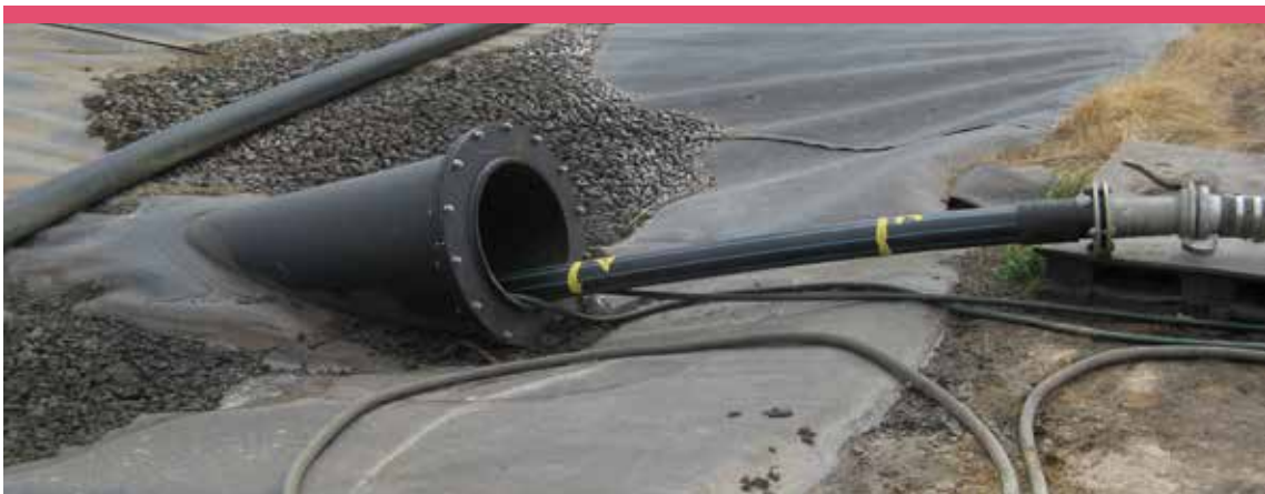
Photograph 7 Pipe threaded through sludge extraction port
