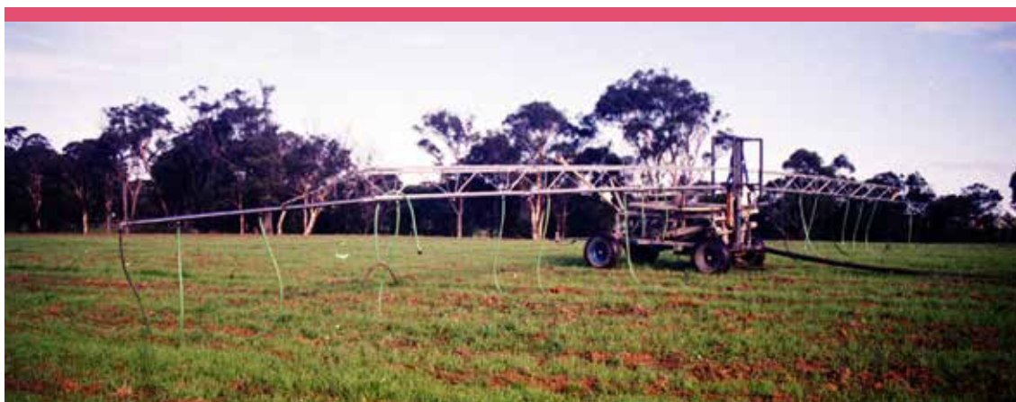
Photograph 5 Dropper irrigators can apply effluent at low rates
