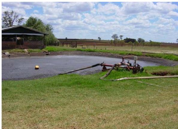
Figure 1 – Sludge removal via pumping
