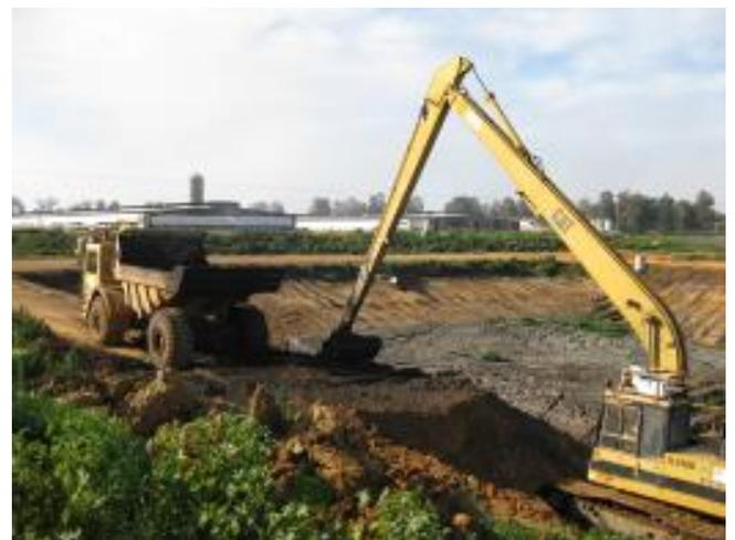
Figure 6 – Excavator removing sludge from a clay lined pond
