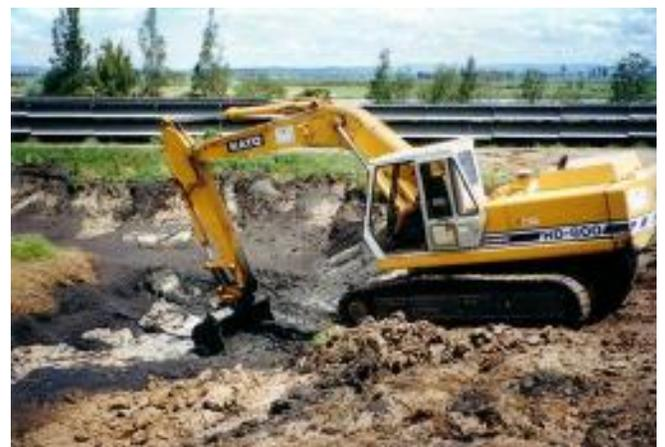
Figure 2 – Mechanical sludge removal from a dewatered pond
