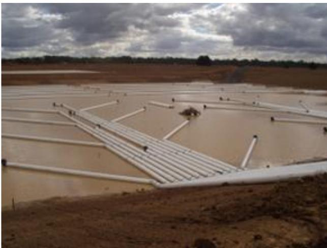
**Figure 7 – Installation of sludge removal pipeline system**
