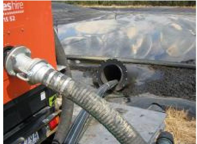
**Figure 9 – Pump suction pipe into a pre-installed desludging pipeline**
