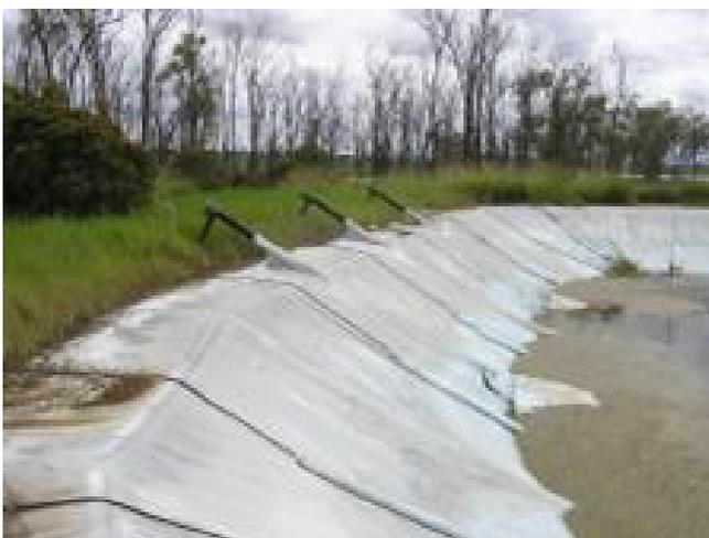
**Figure 8 – Sludge extraction pipelines (deflated pond cover)**
