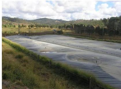
**Figure 3: Covered Anaerobic Pond (above) and Biogas Generator (below)**
