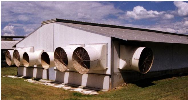
**Figure 2: Tunnel Ventilation System – Exhaust Fans**
