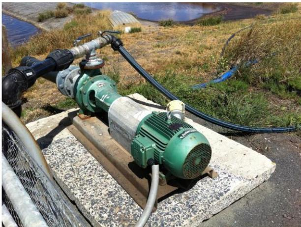
**Figure 5: Recirculation Pump Used to Recycle Piggery Effluent**
