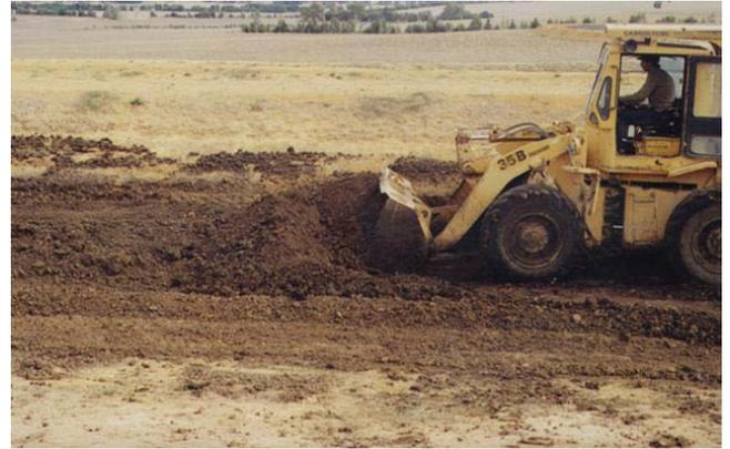
**Figure 4 – Solids removal from dried SEPS bay**
