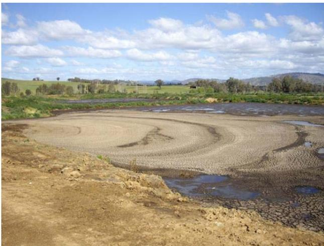
Figure 1 – Long-term sludge drying bay
