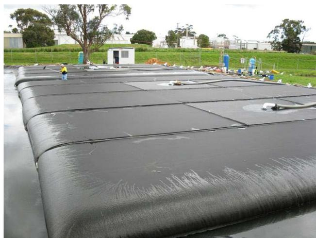
**Figure 6 – Dewatering sludge using geotextile tubes (Dredging Solutions)**
