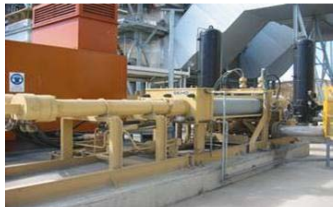
Figure 8 – GEHO DHC valve operated hydraulic piston pump
